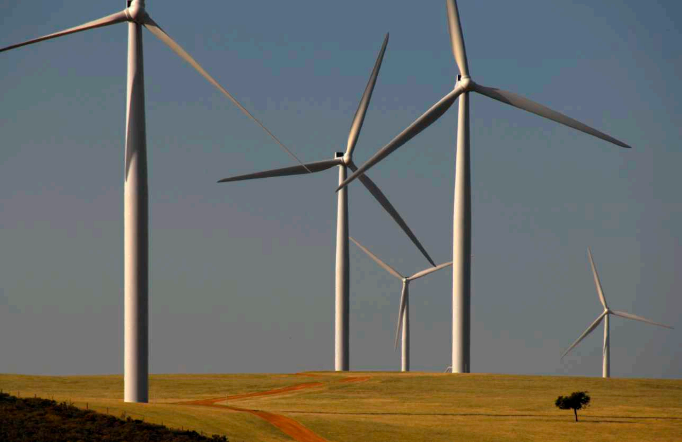
Wind turbines at the Emu Downs Wind Farm, Badgingarra.
